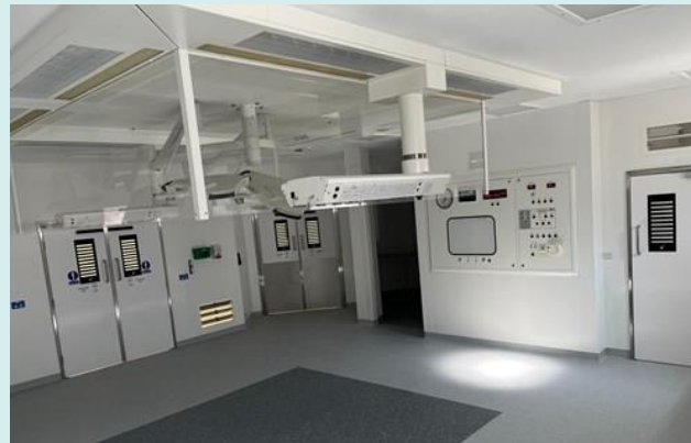
Theatre refurb at Spire Washington Hospital
